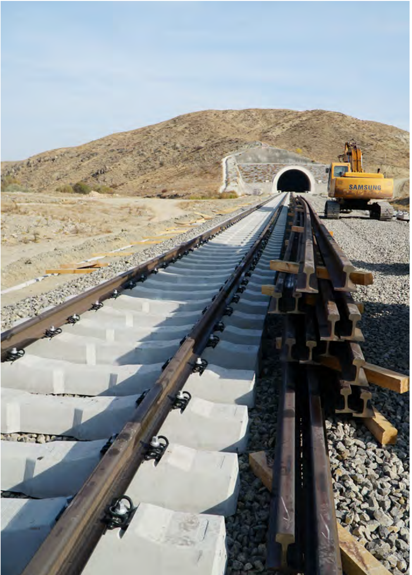
Installation of under sleeper pads Ankara-Sivas
