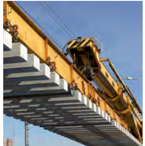
Installation train with turnout padding
