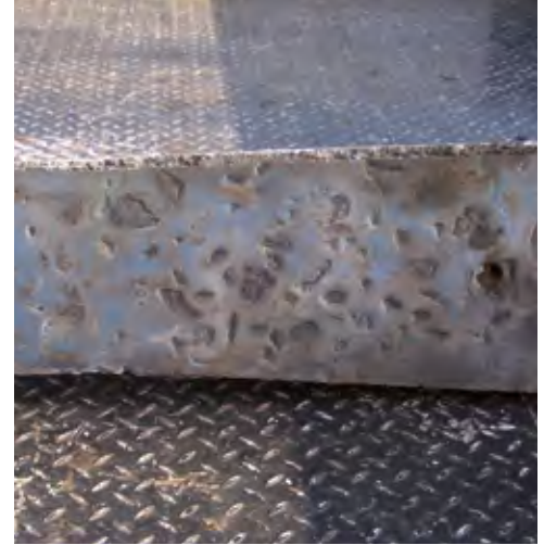
Getzner padding SLB 2210G after 190 million total tons. The plastic impressions in the material prevent shifting by the top ballast layer. No cracks or perforations can be seen in the padding.
