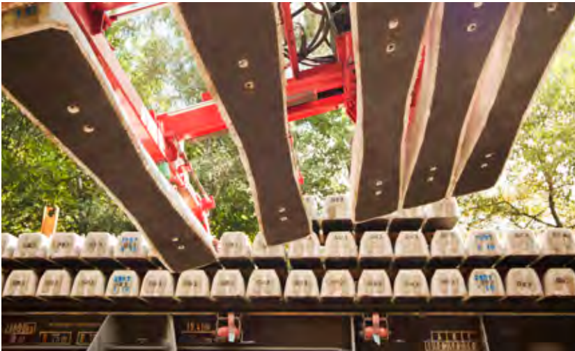
Installation of under sleeper pads on the Berlin-Cottbus ABS
