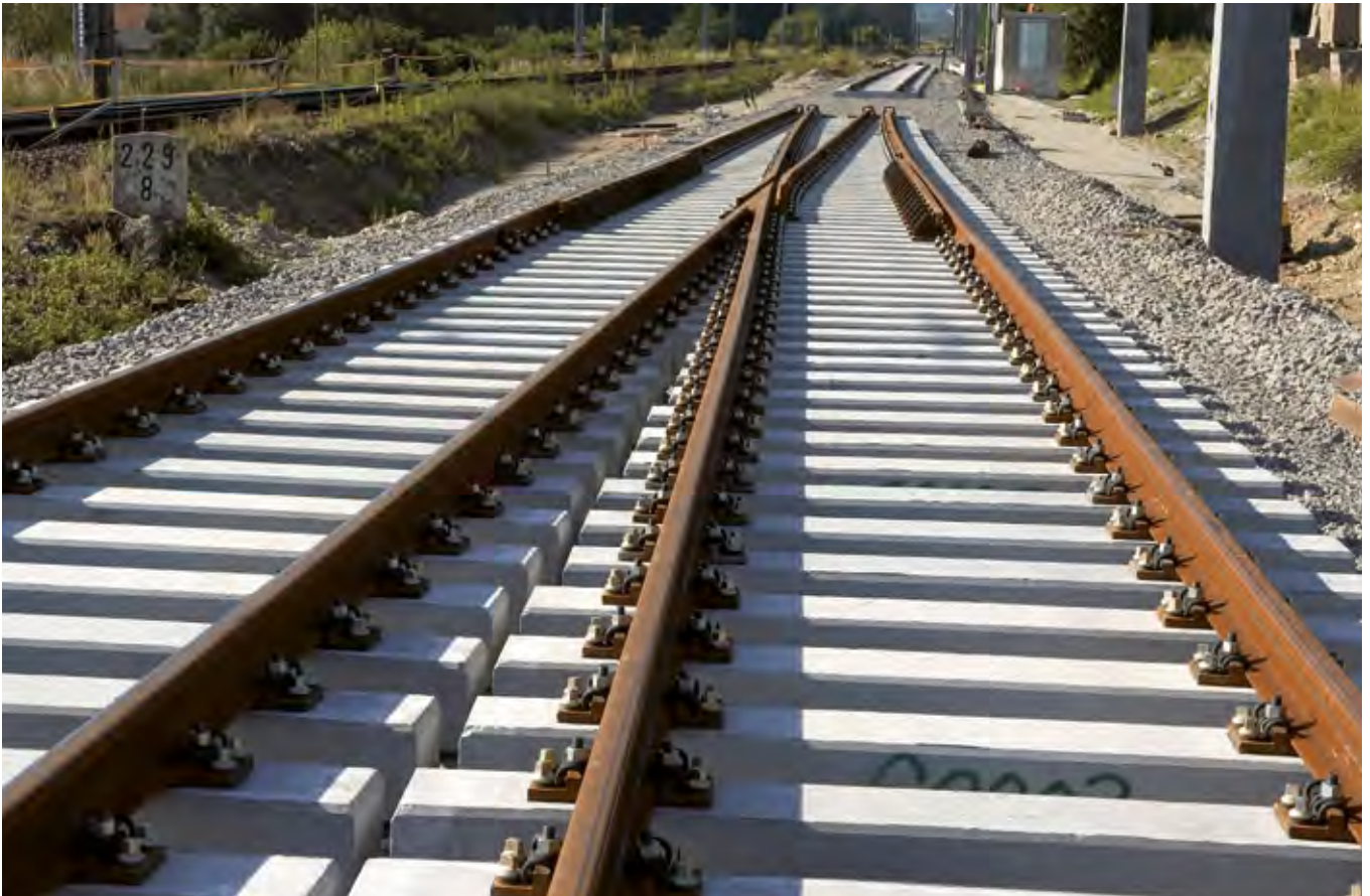
Installation of padded sleepers
